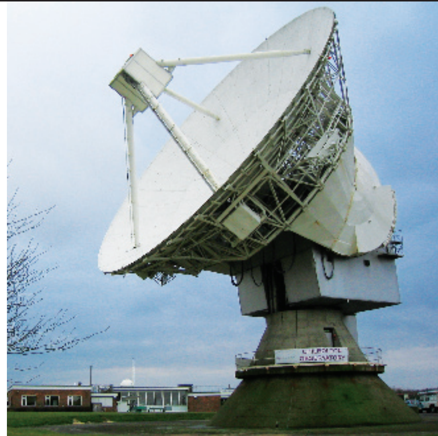
The 25-meter antenna at the Chilbolton Observatory of the Rutherford Appleton Laboratory near Didcot, United Kingdom, used to track GIOVE-A transmissions.
